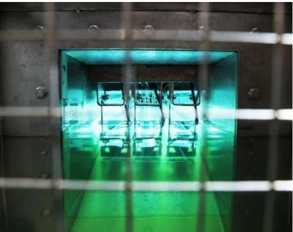
Figure 5: Inlet featuring three module system submerged in stainless steel channel
